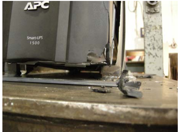
Damage to the Front Panel
