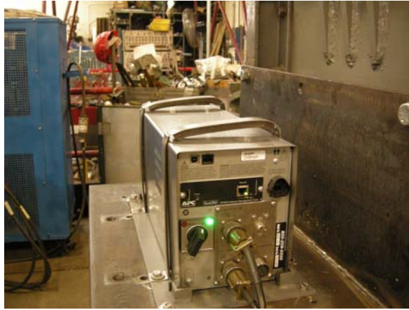
Post-Blow #2, Bent Top Brackets Figure 2
