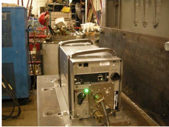
Post-Blow #2, Bent Top Brackets Figure 2
